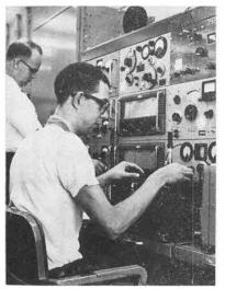
DICK McKNIGHT of AC and RF Standards Section 2412-1 checks a termination (a high frequency resistor) for frequency response over a wide frequency band. At left is Stan Booker, also of Section 2412-1.
